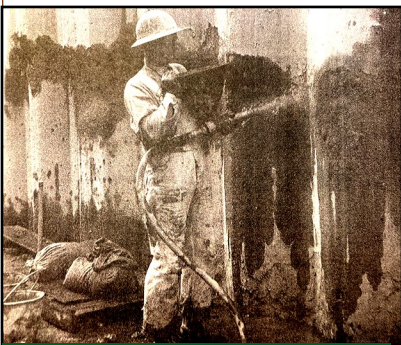
Feb.1942 - Arnold Linde with shotcrete gun.
